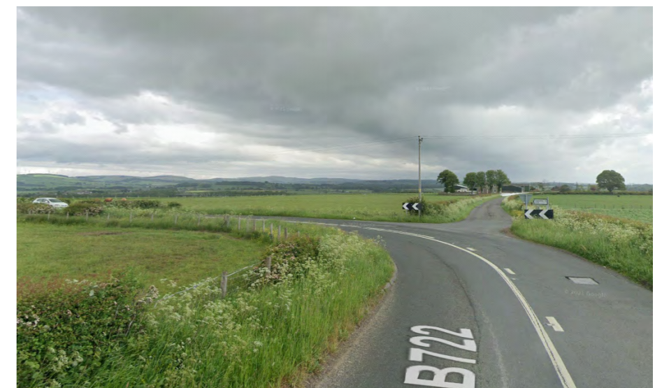
Breaconbeds bend between the site and the A74(M) may require improvement to address issues of visibility and road safety for HGVs.
